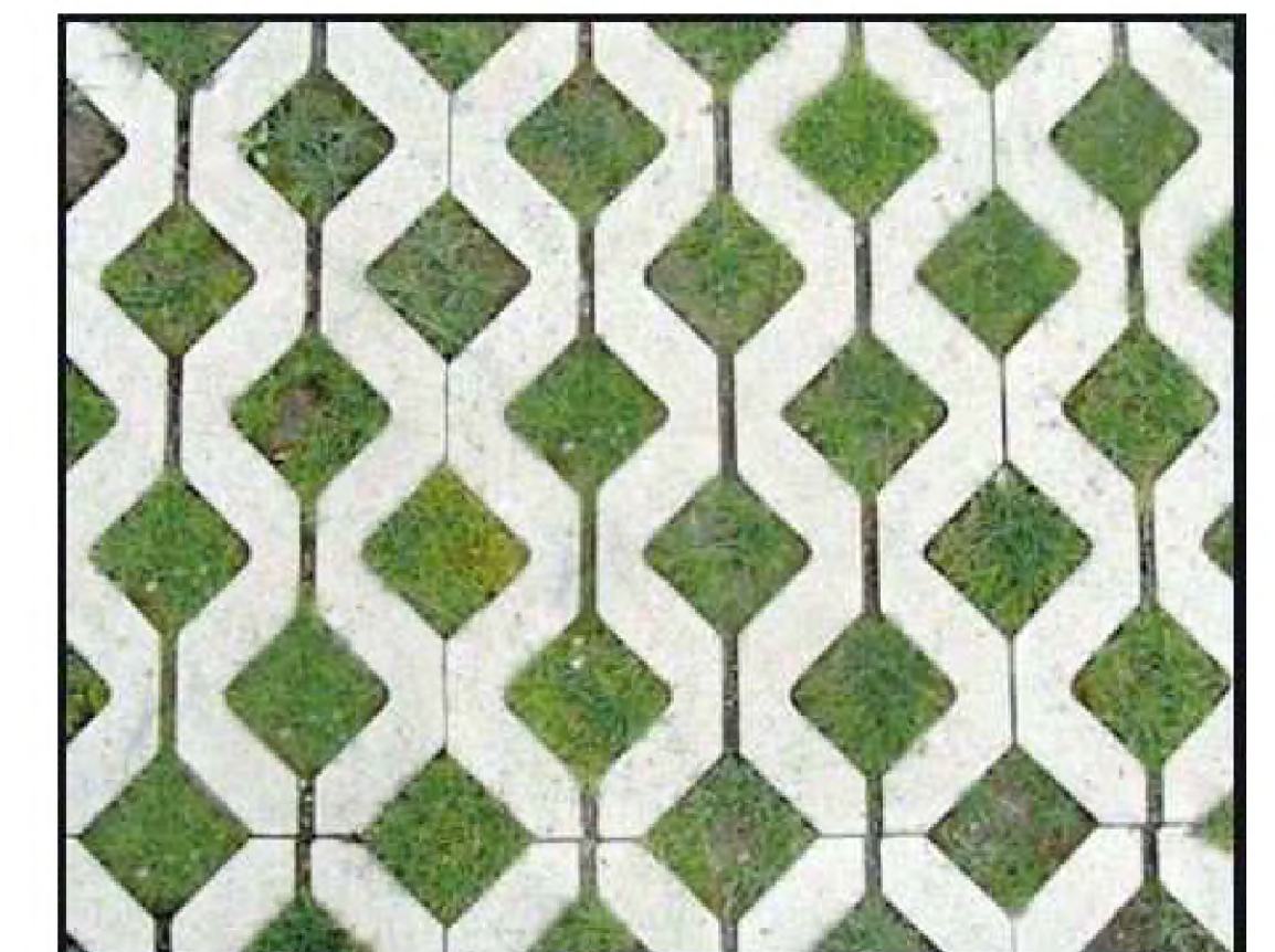
permeable ground works
